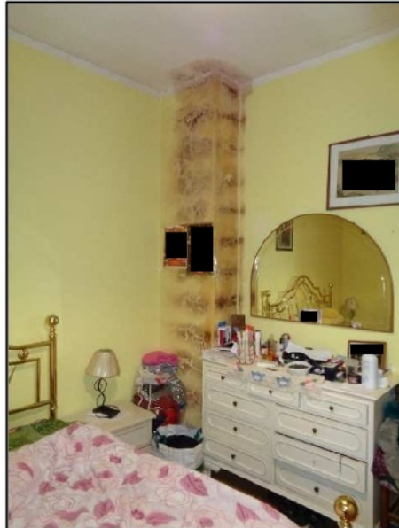
FOTO 19 – CONDENSE/MUFFE CAMERA
