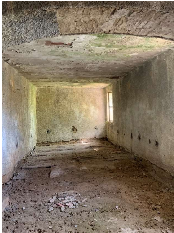
locale al Piano seminterrato
